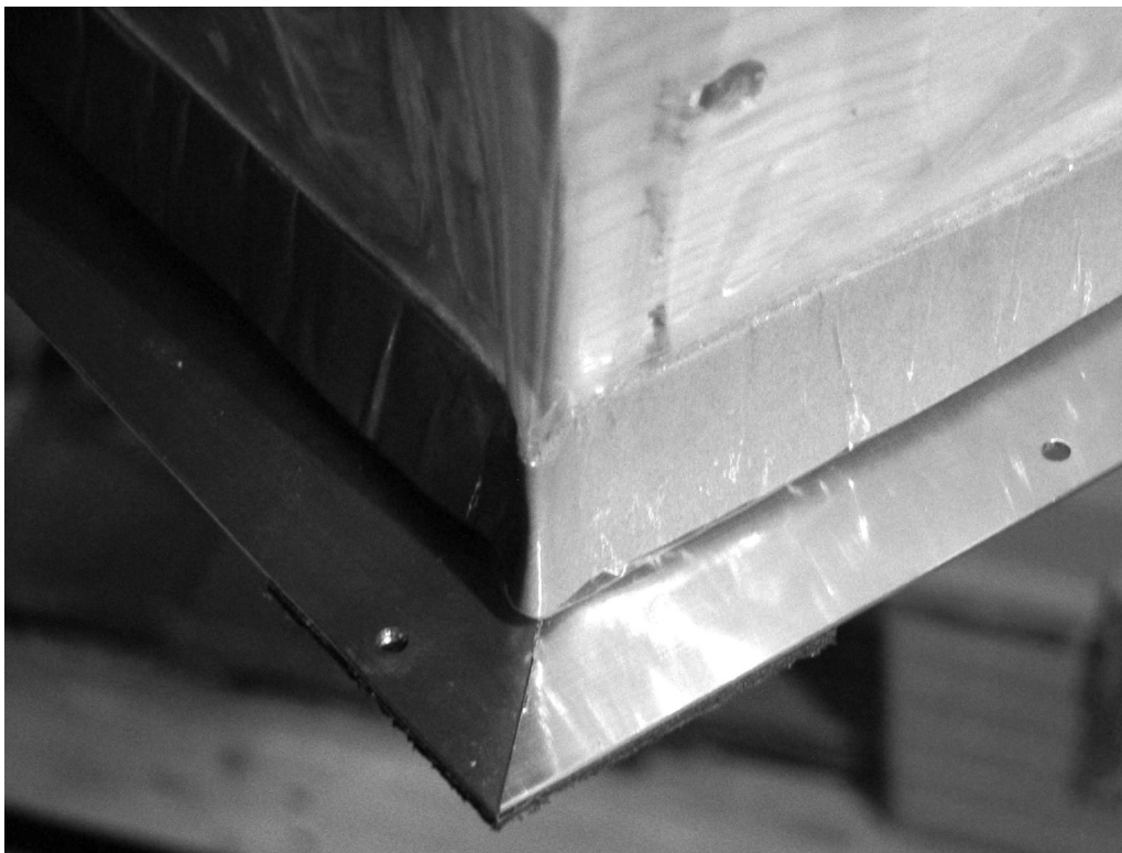
FIG. A1.7 Type B Material Applied to Window Frame
