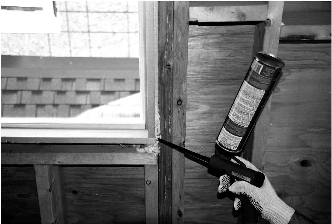
FIG. A1.1 Application of Aerosol Foam Sealant (Type A Material) In Cavity Between Window Frame and Rough Opening
